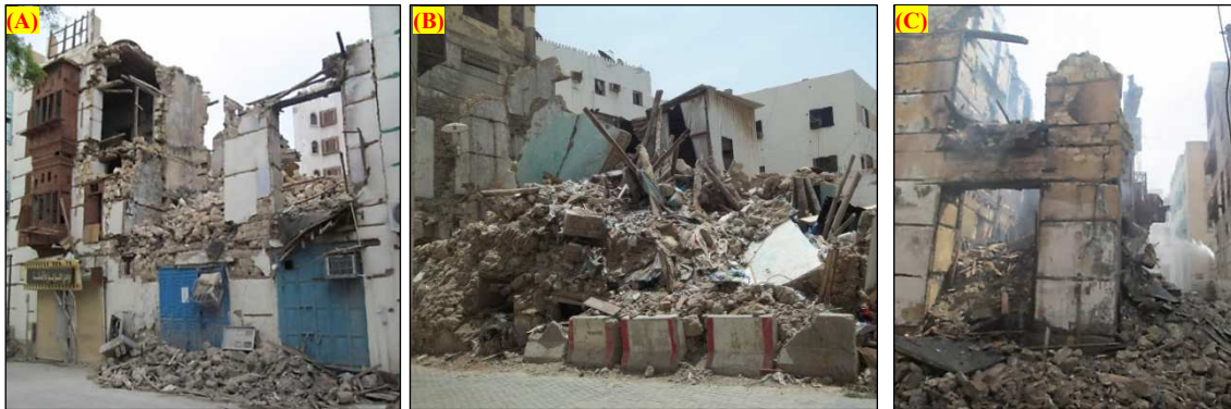
Figure. 15: Failure and collapse of some heritage buildings; (A) Partial collapse; (B): Total collapse; (C) Partial collapse caused by fires.
